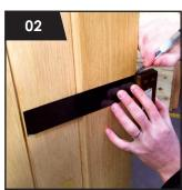
Measure and mark the door handle height. One metre from floor level is typical.
