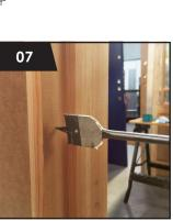
Using the 32mm Spade bit, place the point in the mark on the frame. Drill out the frame to the depth indicated on the spade bit.
