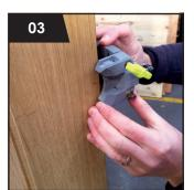
Adjust the backset on the jig to suit tubular latch specification -45mm or 57mm.
