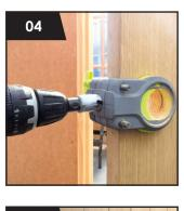
Fit the 25mm hole saw and arbor. Ensuring the drill is level, bore out the latch hole.
