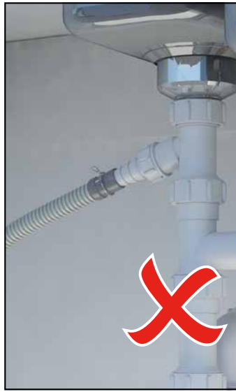
Incorrect waste pipe configuration.
