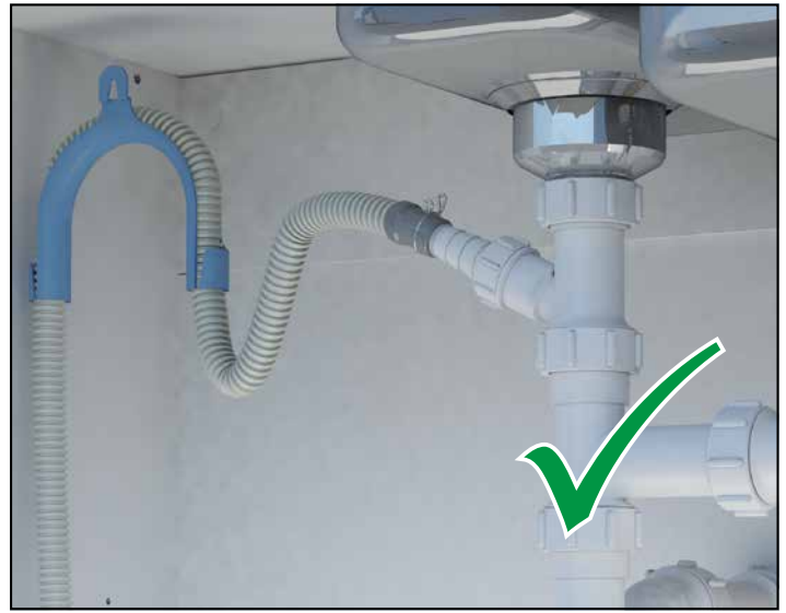
Correct waste pipe configuration.
