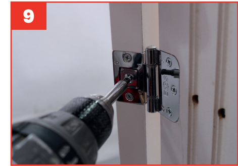
Re-secure the cams back onto the hinges. set cam pin to '0'
