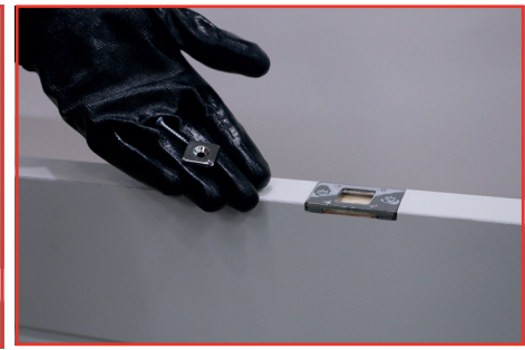
Take the door provided and remove the screws and cams from each of the pre-fitted female hinges. Hinges are Pre-fitted for RH applications. Remove hinge and turn round.
