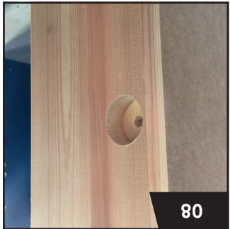
Clear the debris from the hole.
