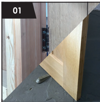
Ensure door is hung and wedged securely.
