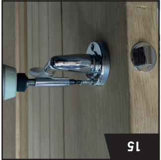
Connect the remaining handle by pushing the sleeves together securely. Fit the 2 machine screws until tight.
