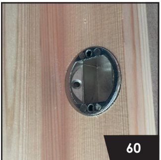
Check the socket fits into the hole, and allows 1mm depth for the striking plate to be fitted.
