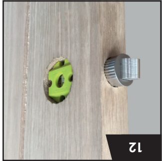
Place the spacer in the handle bore hole. Check for correct handling. Insert the latch in the latch bore hole. Take care to insert the latch with the bolt in the vertical position using a small piece of wood to protect the latch and door, cover the latch bolt and tap the keep into the door, until the face plate is flush with the door. Take care not to use excessive force to drive the latch in. If in doubt, re drill the latch bore with the 25mm holesaw to increase the hole diameter to prevent timber splitting.
