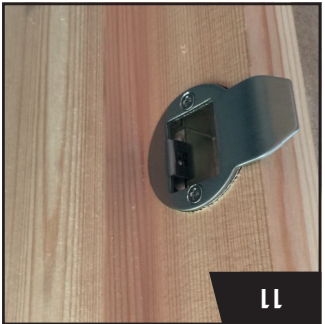
Mark and chisel out for the striking plate lip. Fit the striking plate. Close the door and adjust the anti rattle plates and strike lip to ensure smooth closing action.
