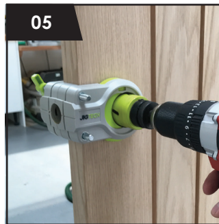
Fit the 44mm hole saw and arbor. Ensuring the drill is level, drill through the guide side of the jig. Withdraw the holesaw to clear debris during drilling. Once the drill tip exits the door on the opposite face remove the jig. TIP: reset the jig by clearing debris from the threads and winding it back to the fully closed position.
