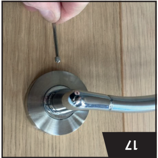
Fit the cover rose in place. Secure with the grub screw provided.
